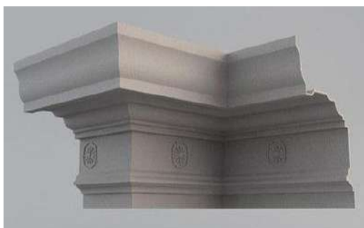
Figure 45 Surgical treatment of facade with the use of GRC cement.
